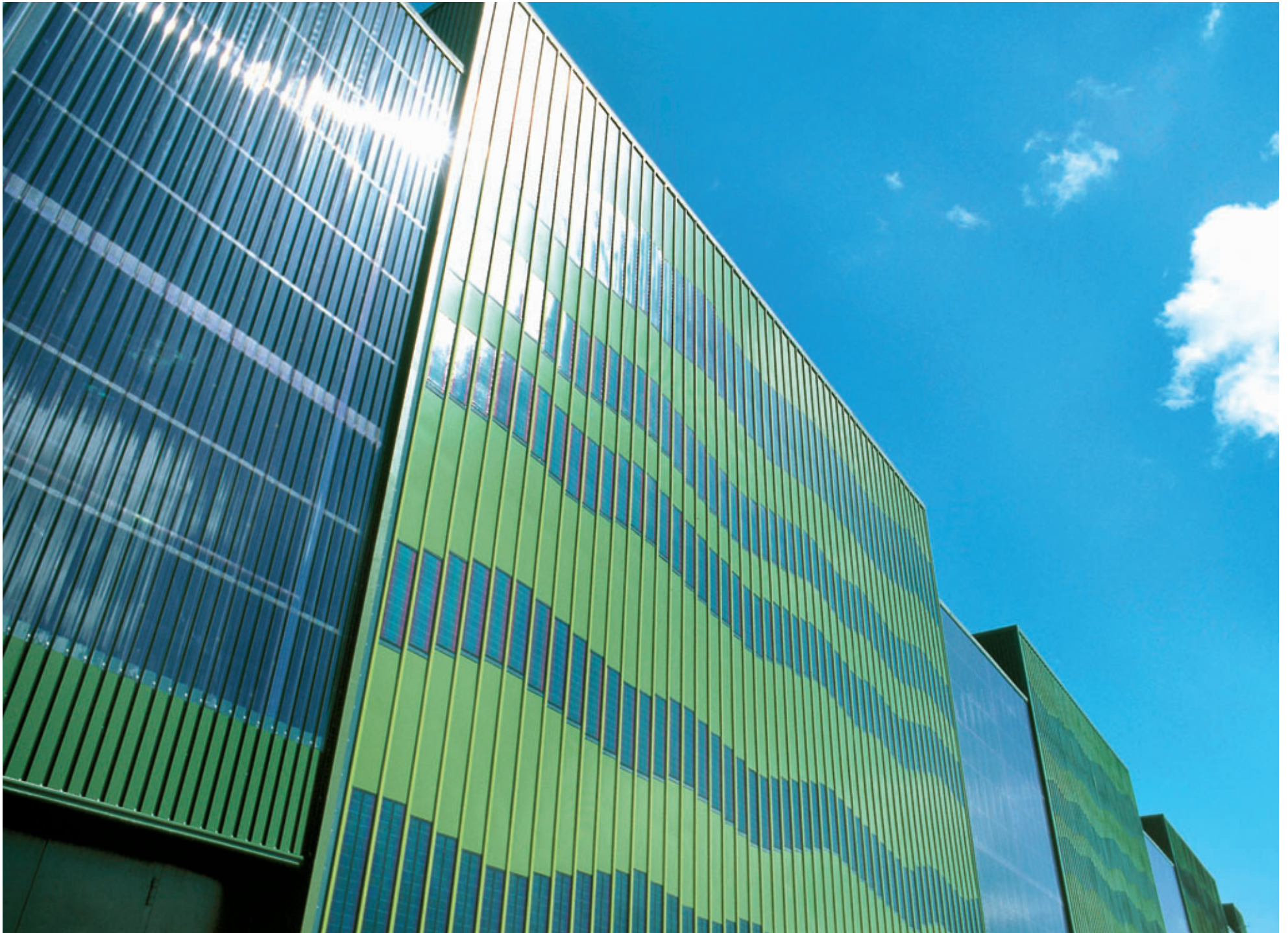
ThyssenKrupp Steel building: Laminated solar foils on steel sheets
